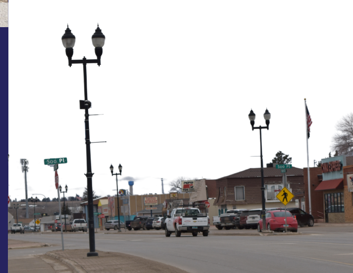
New Town: Main Street Light Project
