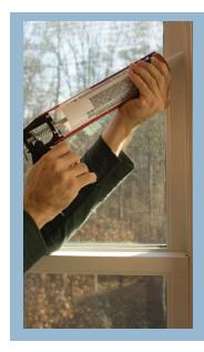
**Keep warm** summer air outside where it belongs! Add caulk or weather stripping to seal air leaks around leaky doors and windows.
